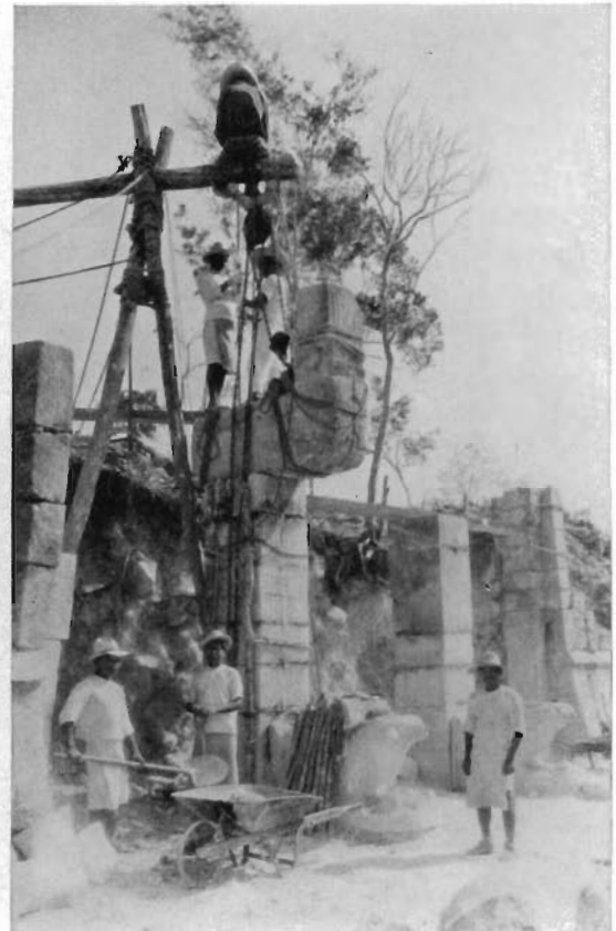
FIG. 61—NORTH SERPENT COLUMN BEING DRILLED TO RECEIVE ANCHOR BOLT
