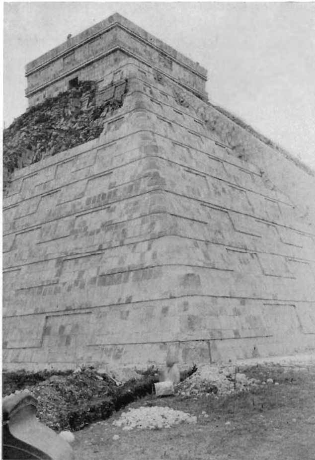
FIG. 50—NORTHWEST CORNER OF CASTILLO AS REPAIRED BY MEXICAN GOVERNMENT
