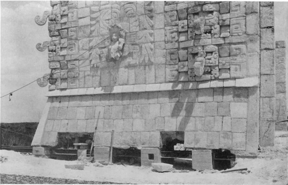
FIG. 89—NORTH ANTA, I-BEAMS OF FOUNDATION IN PLACE
