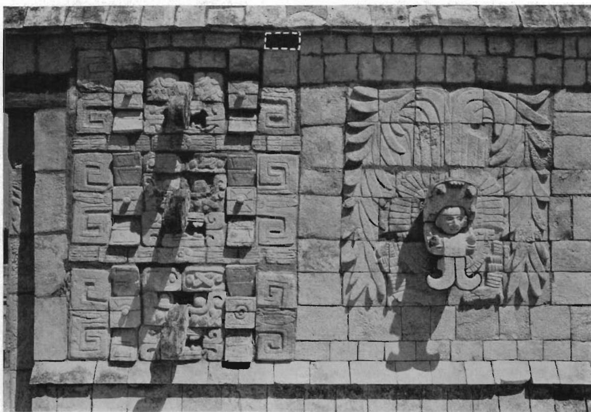
FIG. 17—NORTH PANEL OF MASKS AND PLUMED SERPENT SHIELD, SOUTH ANTA, TEMPLE OF THE WARRIORS Portions outlined in black, made of cement; in dotted-white, of stone, to replace missing originals
