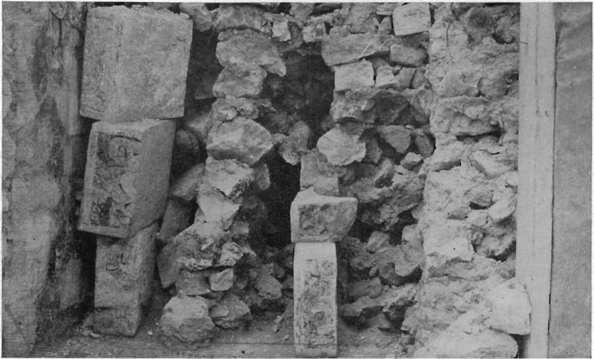
FIG. 87—COLUMN BLOCKS REUSED IN FILL BETWEEN COLUMN 2 AND PARTITION, TEMPLE OF THE CHAC MOOL
