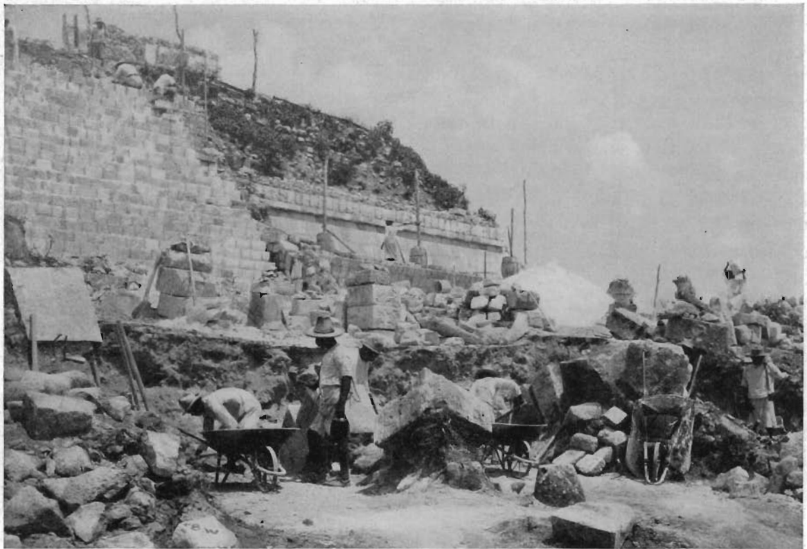
FIG. 72—EXCAVATING TOWARD FOOT OF WARRIORS STAIRWAY
