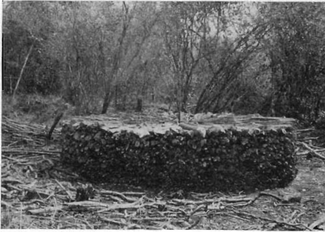
FIG. 133—CYLINDER OF WOOD FOR LIME BURNING, HALF BUILT
