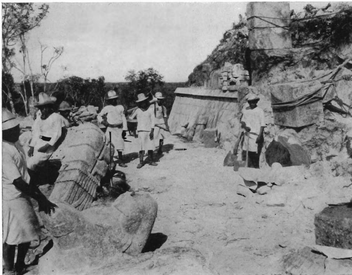
FIG. 59—NORTH SERPENT COLUMN, SHOWING POSITION IN WHICH IT FELL
