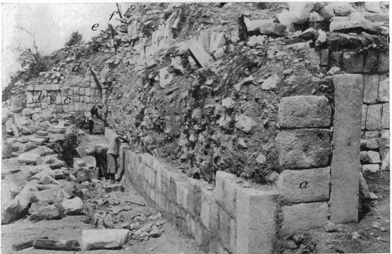
FIG. 77—LOOKING NORTH ALONG BACK WALL OF NORTHWEST COLONNADE DURING REPAIR
