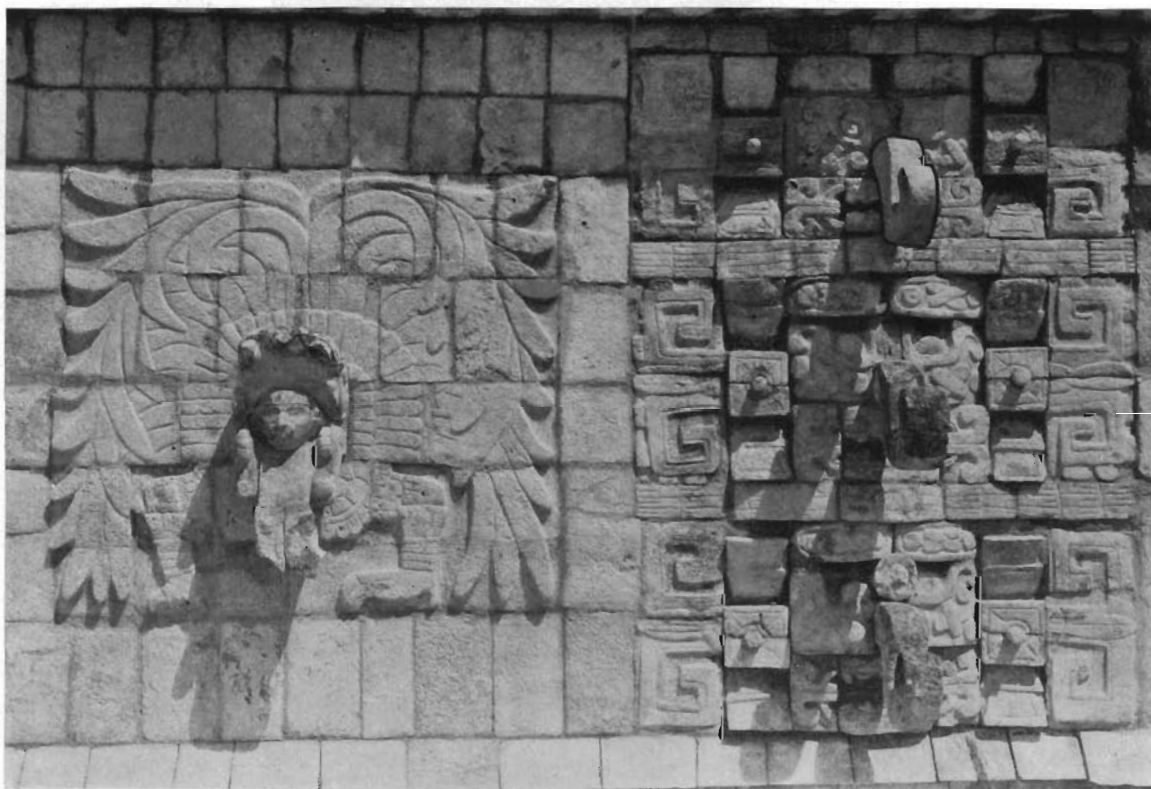
FIG. 9.—PLUMED SERPENT SHIELD AND SOUTH PANEL OF MASK, NORTH ANTA, TEMPLE OF THE WARRIORS Portion bordered with black line, made of cement, to replace missing original
