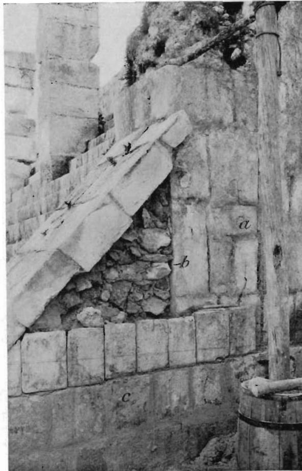
FIG. 40—SOUTH FACE OF STAIR RAMP SHOWING ORIGINAL FACING
