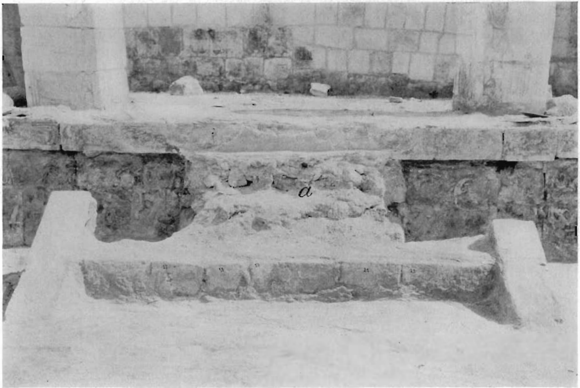
FIG. 39—SECONDARY STAIRWAY IN FRONT OF SCULPTURED DAIS, NORTHWEST COLONNADE, PARTIALLY REMOVED, SHOWING REMAINS OF EARLIER STAIRWAY, a
