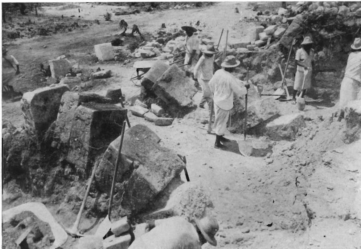
FIG. 79—FRONT OF NORTHWEST COLONNADE SHOWING COLUMNS FALLEN TOWARD THE WEST
