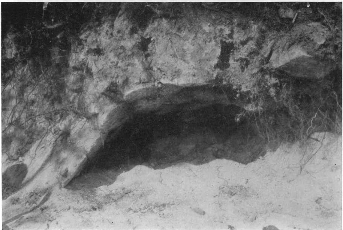
FIG. 65—FALLEN VAULT COURSES IN RELATIVE POSITION
