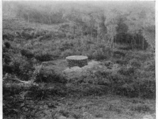
FIG. 134—COMPLETED CYLINDER OF WOOD FOR LIME BURNING
