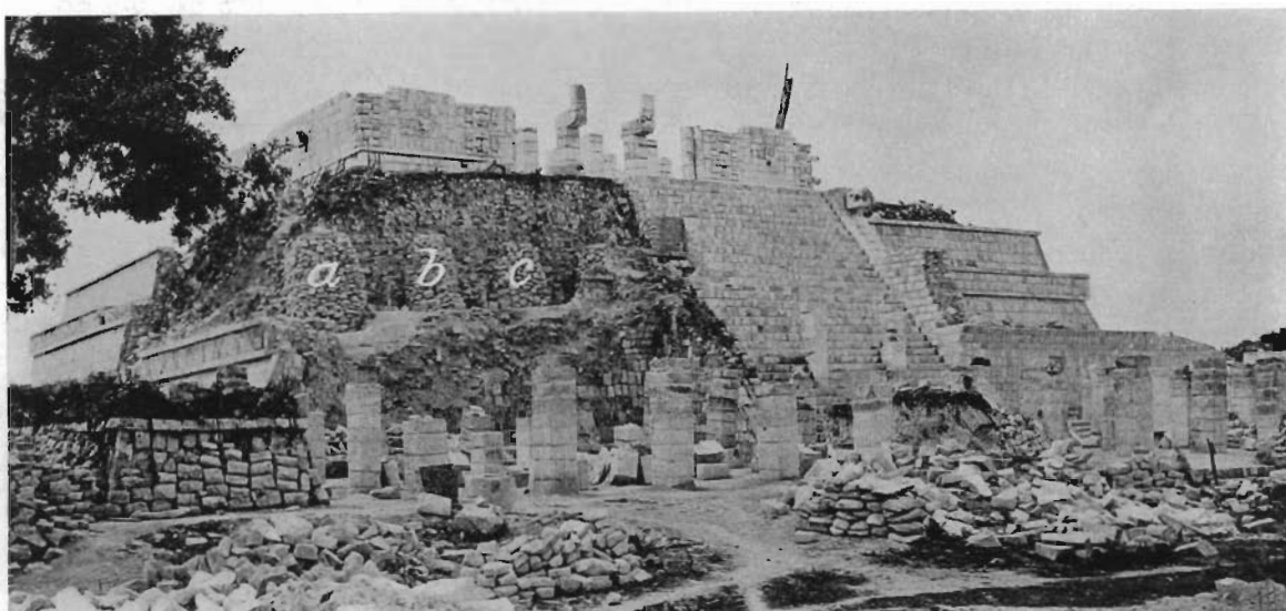
FIG. 84—DRY WALLS BUILT TO ENCLOSE COLUMNS OF TEMPLE OF THE CHAC MOOL
