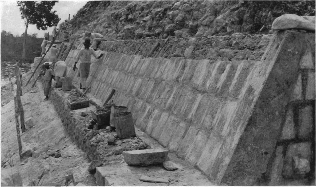
FIG. 126—REPAIRING NORTH SIDE OF PYRAMID
